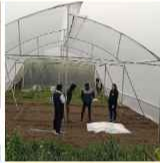
CONSTRUCTION OF POLYHOUSES
