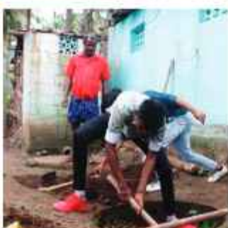
RENOVATION OF TOILETS IN PUTHUPATHE TRIBAL VILLAGE
