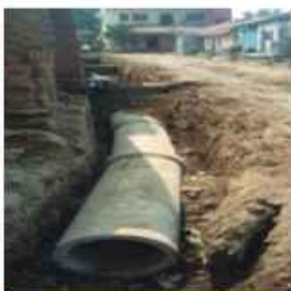
DEVELOPMENT OF UNDERGROUND DRAINAGE SYSTEM
