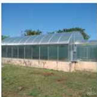
MODEL NURSERY CONSTRUCTION
