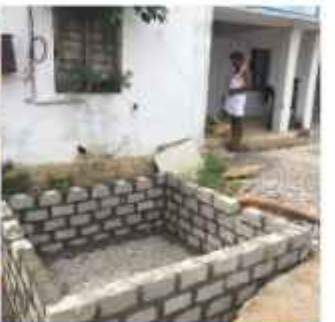
RAIN WATER HARVESTING PITS
